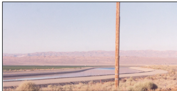
Picture 5.4: California Aqueduct in Kern County
